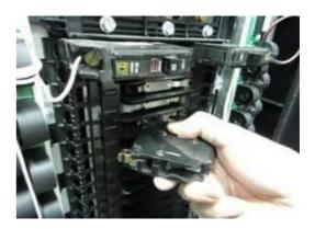
The breakers can be safely add-ons and replace without down time.
