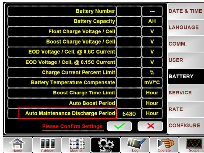
Figure0-4 Setting period for battery auto discharge
